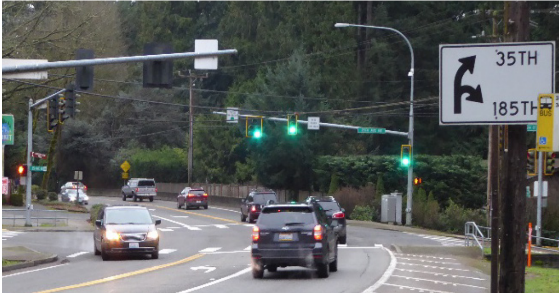
Approach to 35th Ave NE Intersection. Street sign shows the sharp angle of intersection legs.
